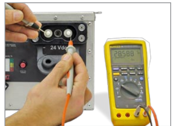
Figure 3.9.3 – Testing DC Receptacle
