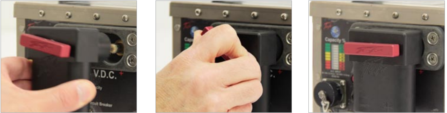
Figure 3.10.1 Attaching DC Power Cable to TI60 MPU-24
