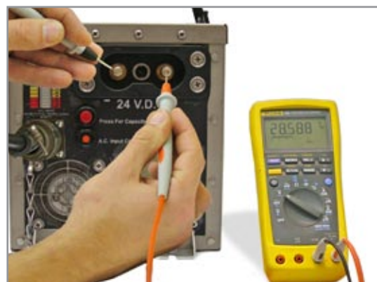
Figure 3.9.3 – Testing DC Receptacle
