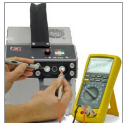
Figure 3.9.3 – Testing DC Receptacle
