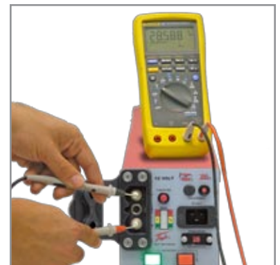
Figure 3.8.3 – Testing DC Receptacle
